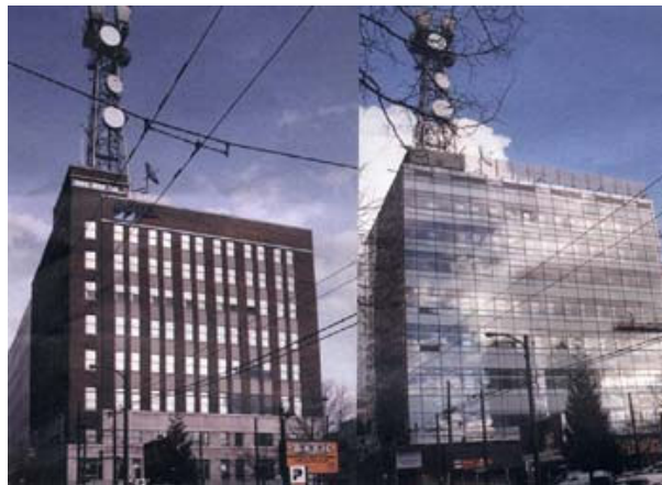
Fig. 11. View Showing the Old and New Facades [1]
