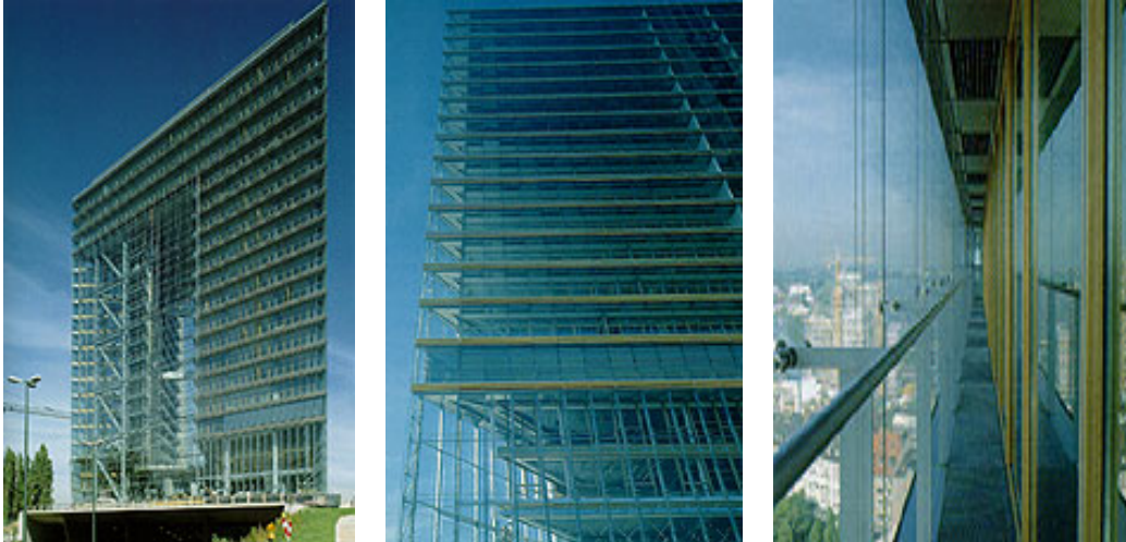
Fig. 13. Photographic Views of the Stadttor Building [17]
