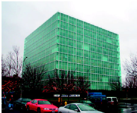
Fig. 8. View of the Hooker Building [5]
