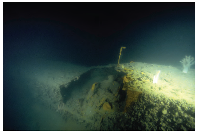
Figure 4. Metal loss on the conning aft of the conning tower showing flash rusting after recent deconcretion: Photo by MarkSpencer.com.au
