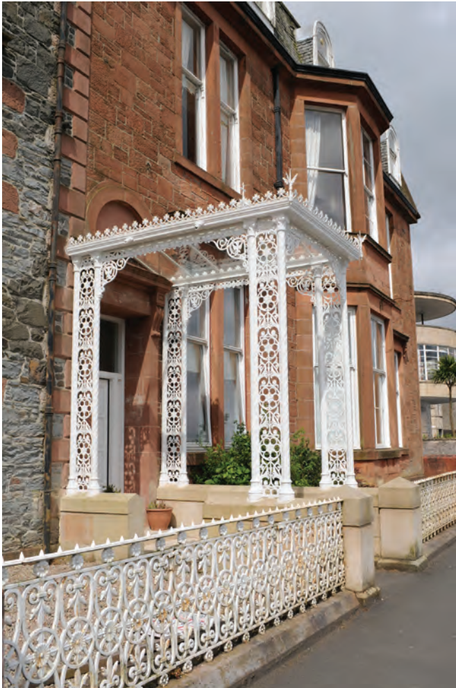
Figure 6. The Bute canopy, June 2009, after conservation
