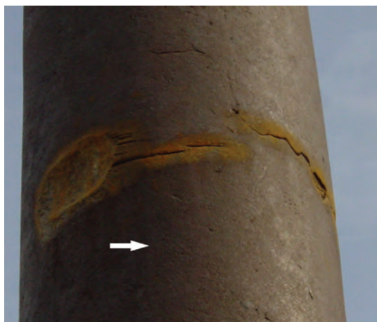
Figure 2. The large dent in the Delhi Iron Pillar. An accumulation of yellow corrosion around the dent and associated cracks is evident. Arrow indicates area where severe pits are noted on the surface.
