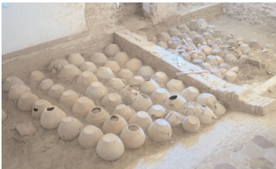
Figure 1. Filling material of the vault.
