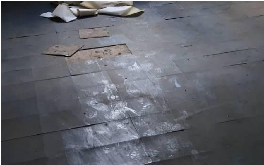
Fig.10. FLOOR IN LINOLEUM TO REMOVE
