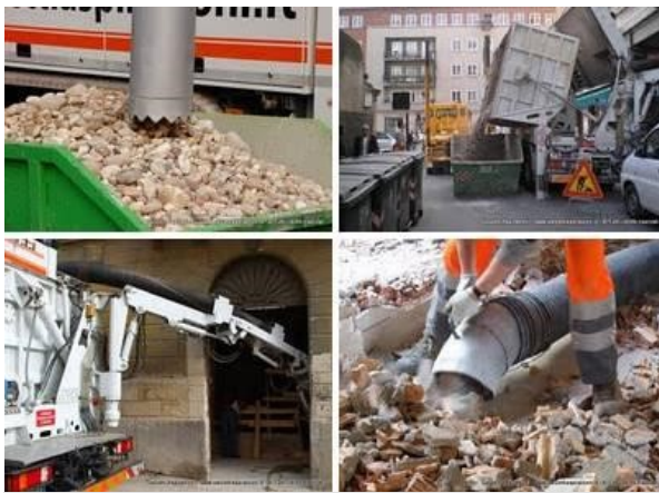
Figure 22. SUCTION MECHANIZED DEBRIS
