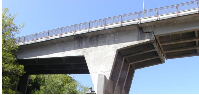
Figure 2.16 Gerber-type system of Belvedere bridge in L'Aquila.
