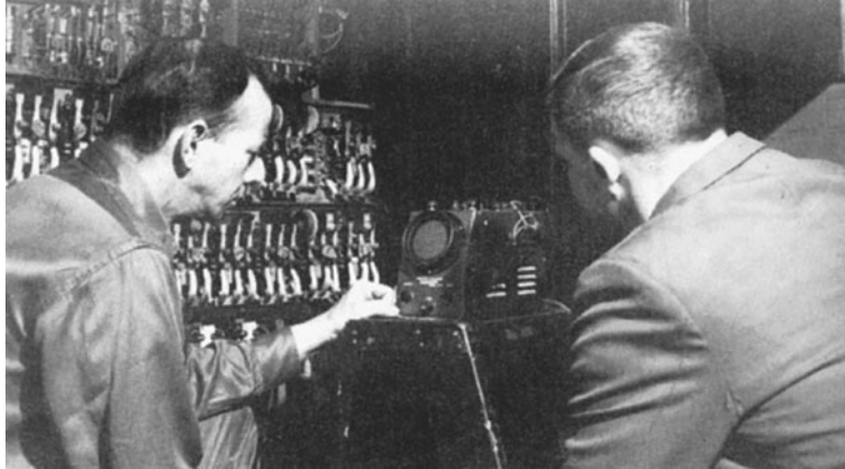
FIGURE 4.2 Cathode-ray-tube oscilloscope typifies the more advanced instruments that maintenance technicians use in analyzing the performance of modern elevator equipment. Checking the operation of automated elevators with great accuracy, the technician can promptly make any necessary adjustments to restore “like-new” service.
