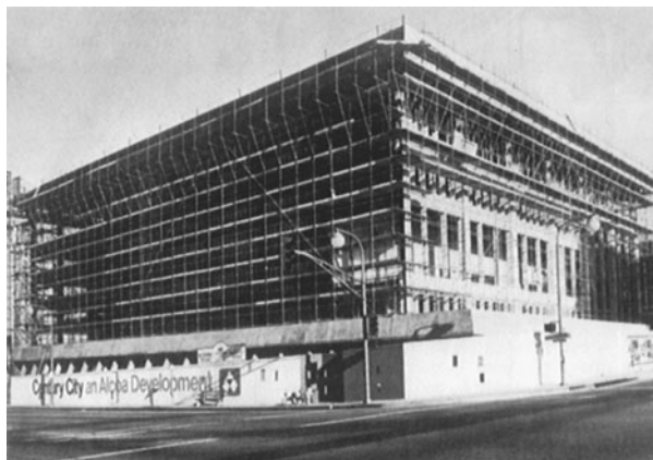
FIGURE 5.9 This shows Tubelox scaffolding used to scaffold building surfaces with a difficult roof-overhang condition. The versatility of Tubelox is similarly utilized for cooling towers, spheres, and refinery structures.
