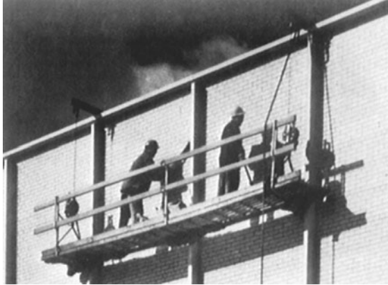
FIGURE 5.8 Safety swinging scaffold (two-point suspension). Utilizes steel-wire rope with ratchet-action raising and crank-handle lowering. Note use of guardrails, midrails, and toeboards. Similar scaffolds are also available with power machines and aluminum platforms. Safety belts, lifelines, and lanyards must always be available and used on all swinging scaffolds.
