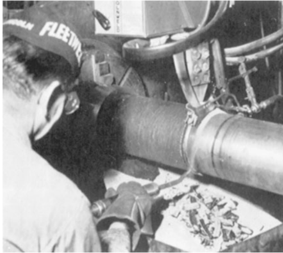
FIGURE 1.44 Submerged arc welding being used to hard-surface a cylindrical surface.
