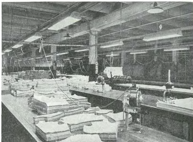
FIG. 143.—Well-arranged fluorescent lighting. (Courtesy of Boris Smoler & Sons.)
