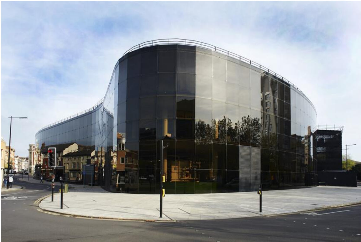
Willis Building in Ipswich one of the first buildings designed by Norman Foster
