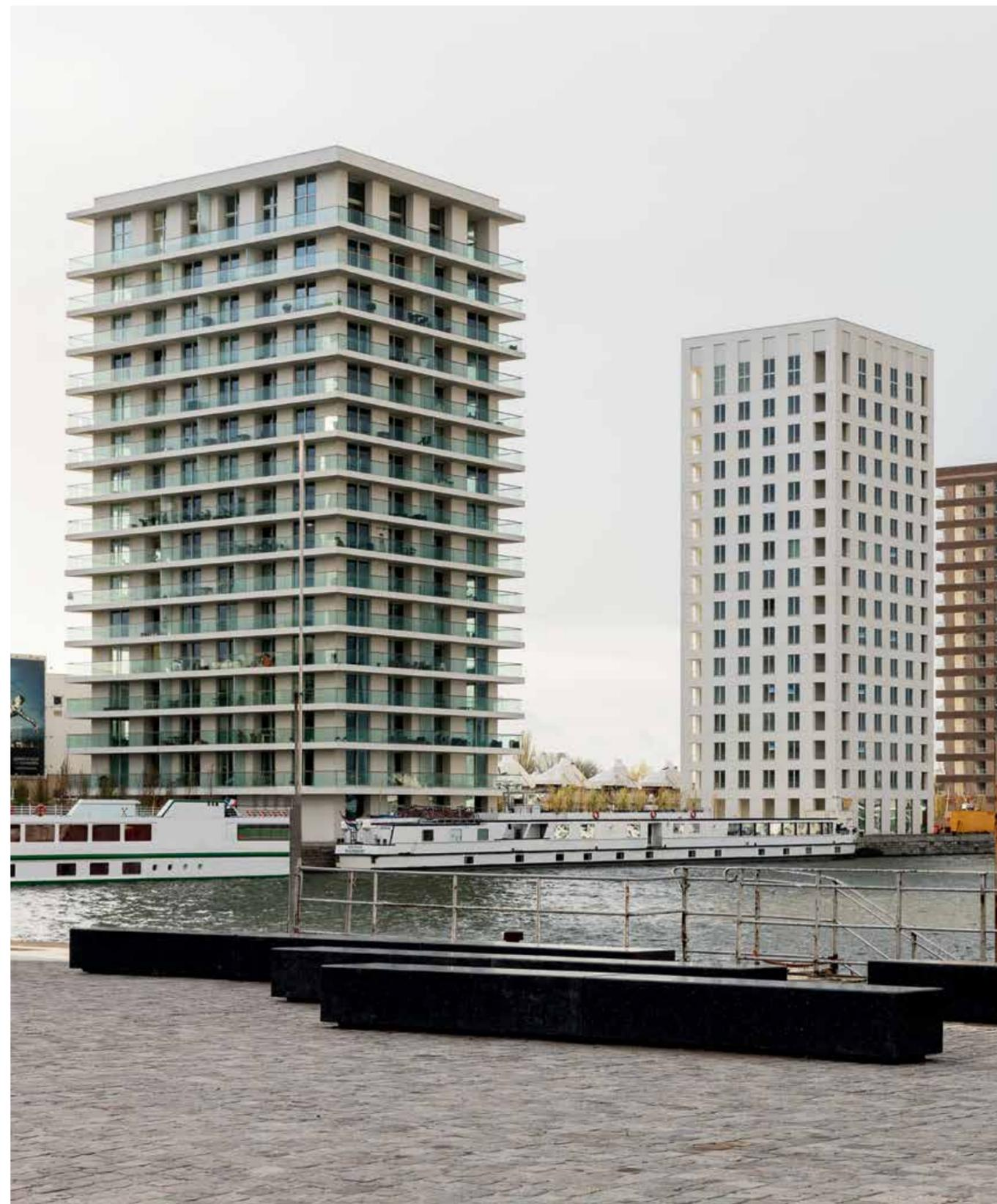
■ Opposite page: tower three is characterised by cantilevered floor slabs all the way up, forming wide balconies wrapping around the building's perimeter and functioning
