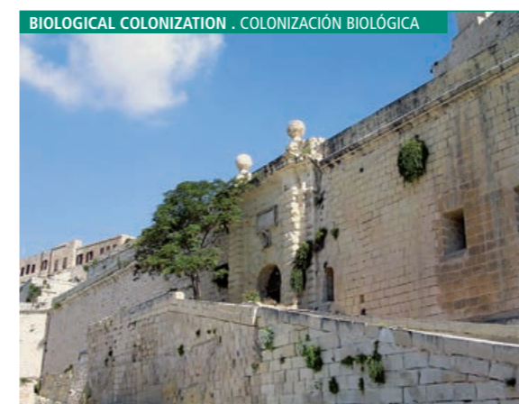
Biological colonization (essentially plants and algae ) on a limestone masonry.
