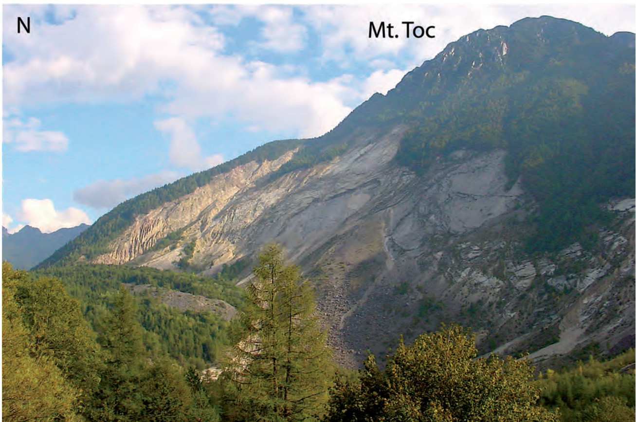
Fig. 1.8 - The landslide from Mt. Toc that generated the Vajont tragedy of the 9th October 1963, in which the water of the underlying artificial lake was squeezed out and devastated the city of Longarone with 1910 casualties. The decoupling surface is the basinal Middle Jurassic Fonzaso Fm, and the dip of the beds is due to the deeper S-verging ramp of the Belluno Thrust.
