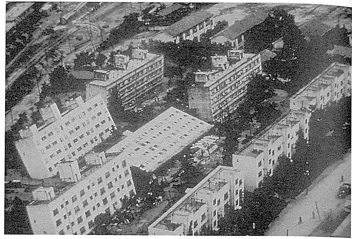
Fig. 1.2-13 Damage to apartment buildings caused by soil liquefaction during the June 16, 1964, Niigata (Japan) earthquake. About a third of the city sank by as much as 2 m as a result of sand compaction. (Courtesy of the National Geophysical Data Center.)
